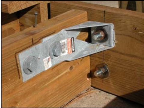
Figure 8 Connector holding post to joist with bolts
