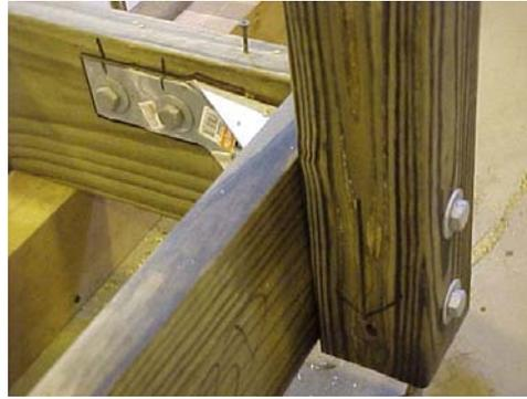
Figure 9 Another view of connection showing post located “outside” the band joist
